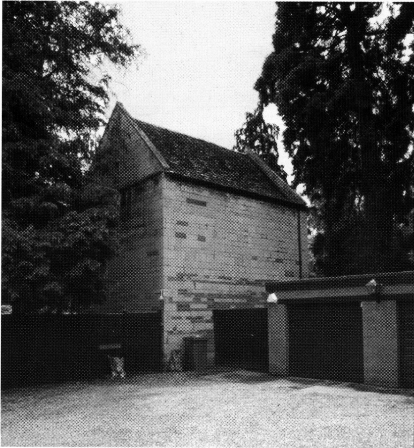
Fig. 2 The dovecote at Water's Edge, Ketton, is wholly of ashlar. Note the perching ledge across the gable
